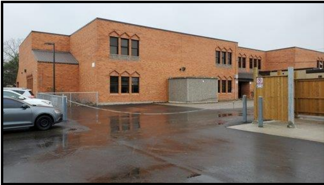
New Parking Lot and New Garbage Enclosure
