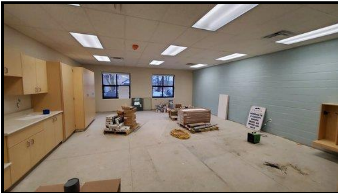
Child Care Room – Under Construction
