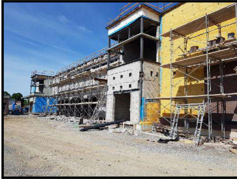
View of east elevation. – June 26, 2018
