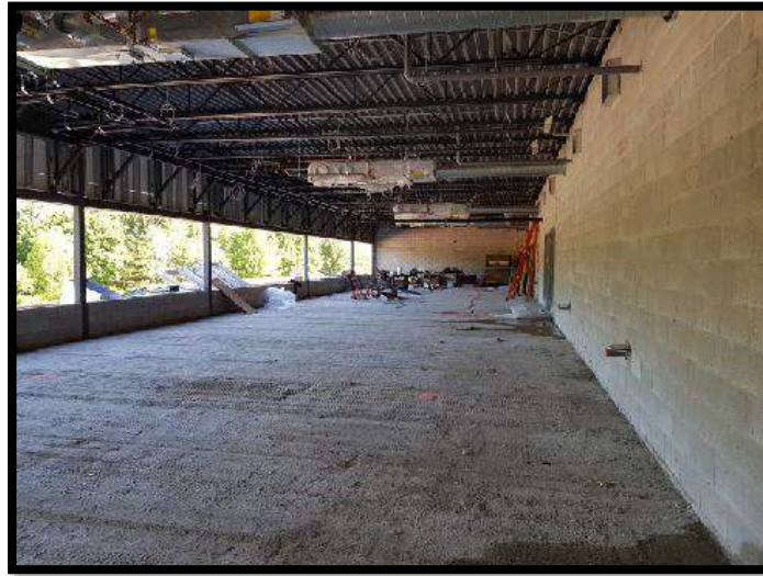
Level 2 classrooms – June 5, 2018
