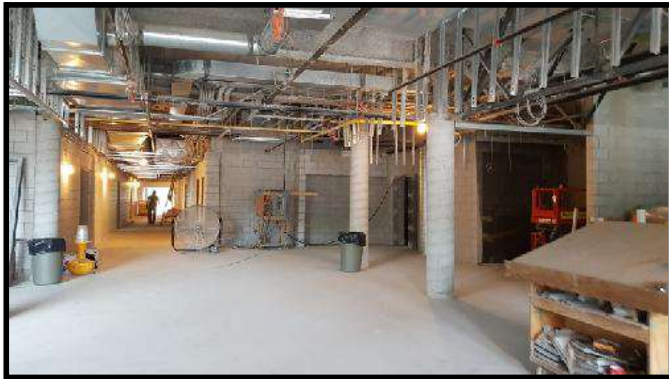
Main entry (foyer) into school
